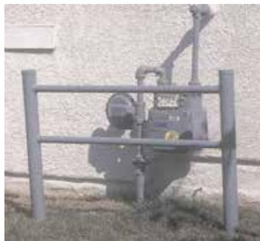
The Industrial Guard Post (left) is a medium duty barrier and the Residential Guard Rail (right) is a light duty barrier. Both are used to protect meter sets and/or regulator stations from vehicular traffic. The above ground portion of both is coated with a minimum of 2.5 mils polyester fusion coating.
